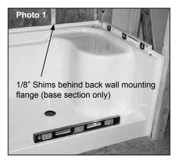
flange at each framing member. Attach the flange across the back first, followed by the ends and then along the front vertical flanges, using 1-1/4" long nails or other appropriate fasteners, approximately 7"-9" apart. Continually check to make sure the base component remains square and plumb within the framed area as it is being secured to ensure proper alignment for the upper sections (photo 2).
